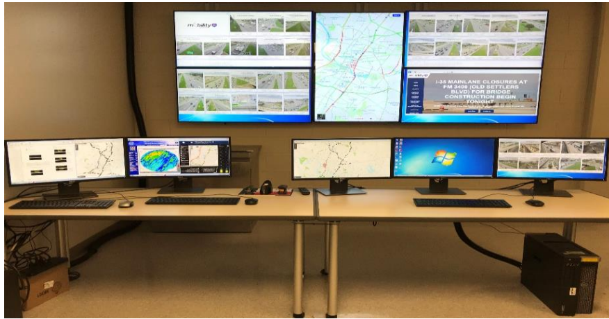
Mobility35 Traveler Information System (TIS) Construction TMC is activated during major construction closures.
